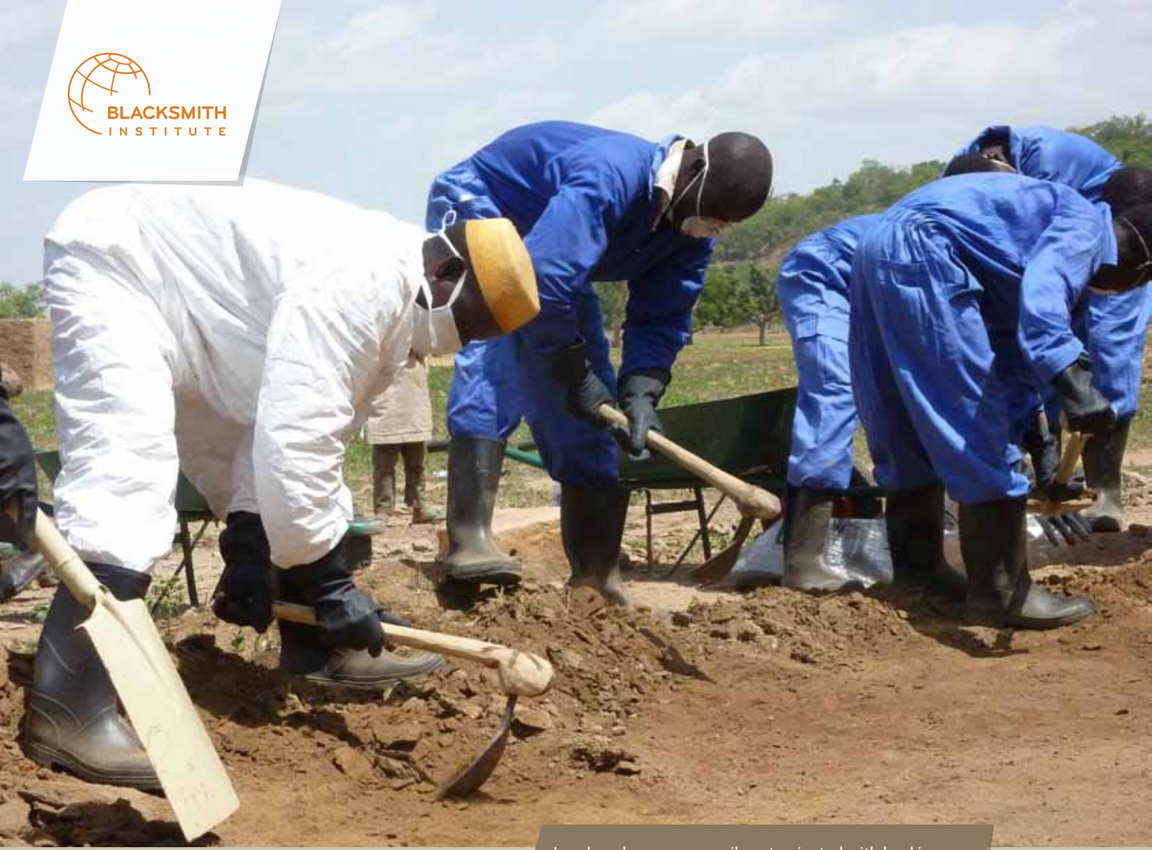
Local workers remove soil contaminated with lead in a village in Northwest Nigeria
