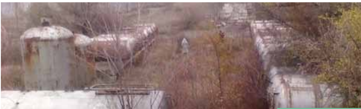
Pesticide storage tanks
