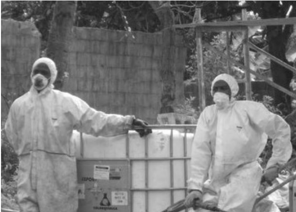
Local contractors in the Dominican Republic were hired and trained to manage hazardous materials cleanup
